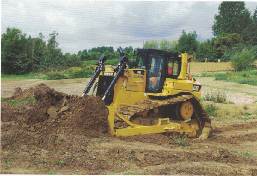
Earthmoving operations at a Cullimore site
